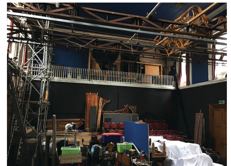
courtroom; the scaffold to the left is currently supporting two failed main roof trusses
