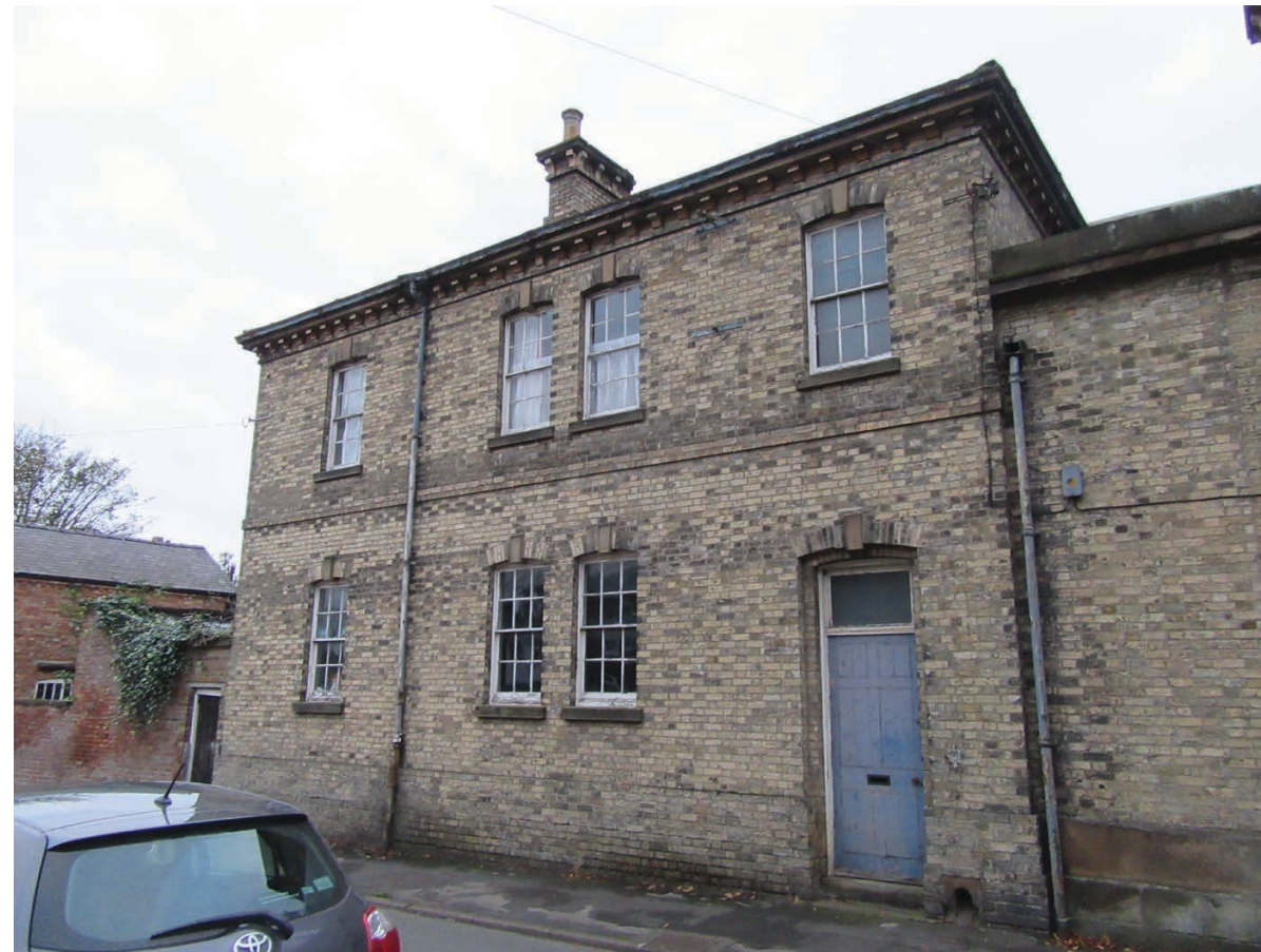
police house, 1870s; the joint in the brickwork between the 1870s and 1820s construction can be seen to the far right of the photograph
